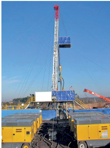
Fig. 5. KREMCO K-600 rig drilling a deep dewatering well [6]
