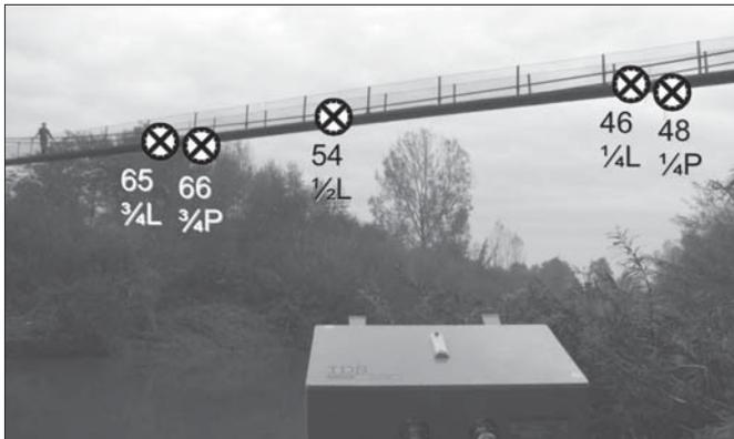
Fig. 4. Arrangement of reflectors on the footbridge
