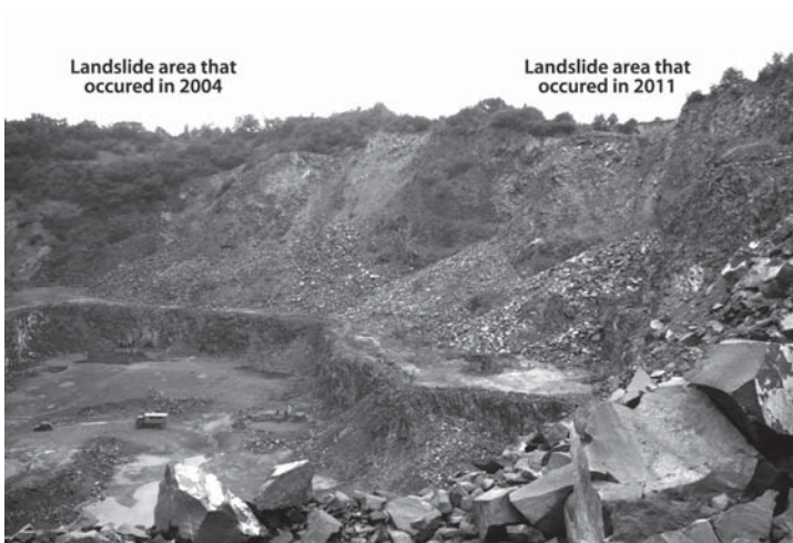
Fig. 3. Open cast view with the marked landslide area in 2004 and 2011
