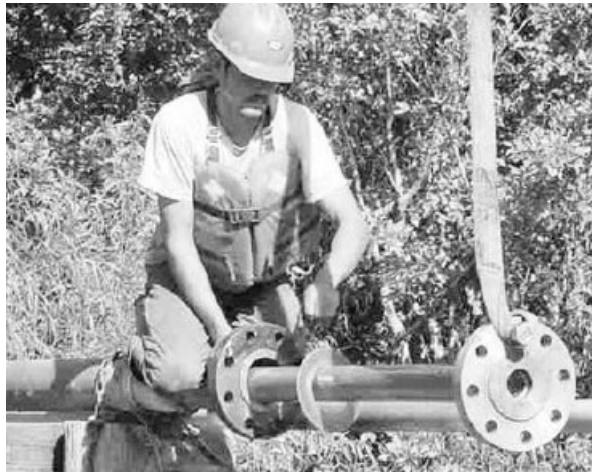
Fig. 4. Application of Thermoflex® pipes for trenchless technology of pipelines modernization
