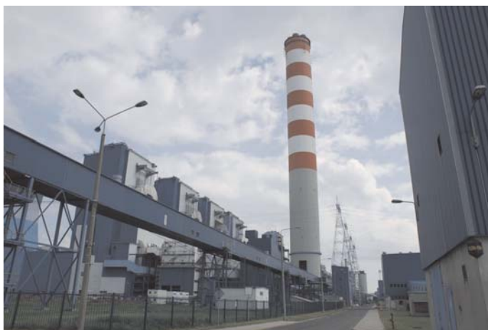
Fig. 6. Experimental facility – cylindrical reinforced concrete industrial chimney of H = 250 m
