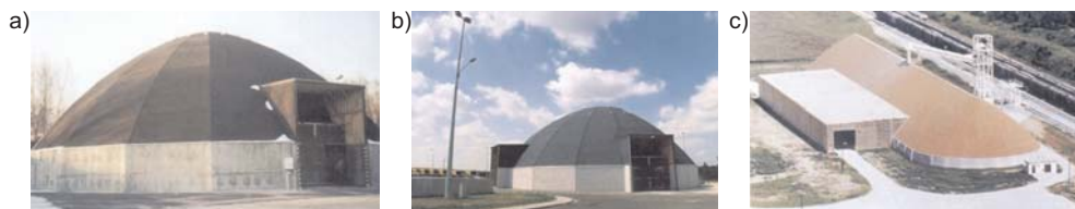
Fig. 1. Types and shapes of warehouses for the storage of loose materials: a) round; b) elliptical; c) barrel-shaped ( http://www.dome-international.com )
