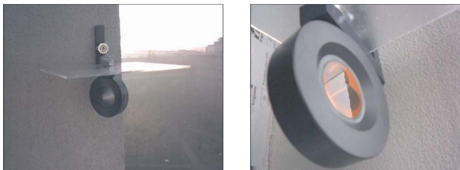
Fig. 2. Exemplary installation of circular prisms
