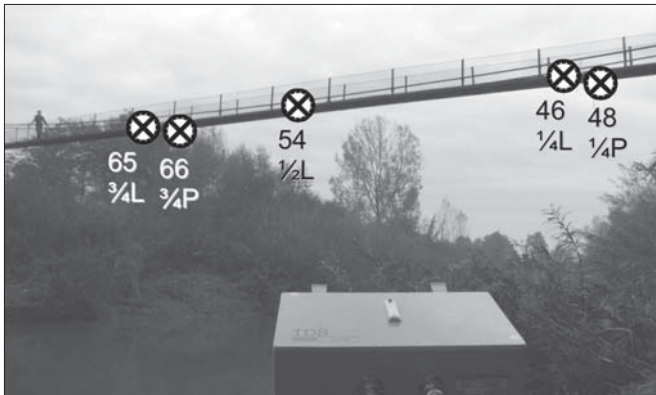
Fig. 4. Arrangement of reflectors on the footbridge
