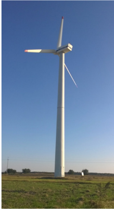
Fig. 1. Examined facility – wind turbine (November 2016 – Kluczewsko, phot. P. Klapa)
