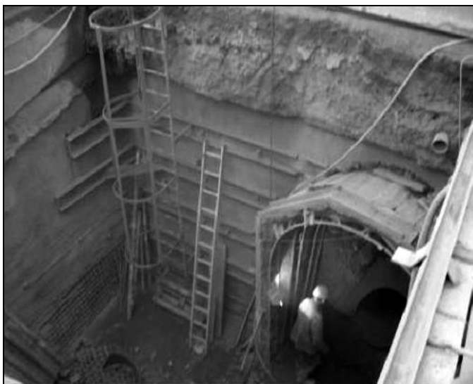
Fig. 3. View on the exit of collector opening before the driving
