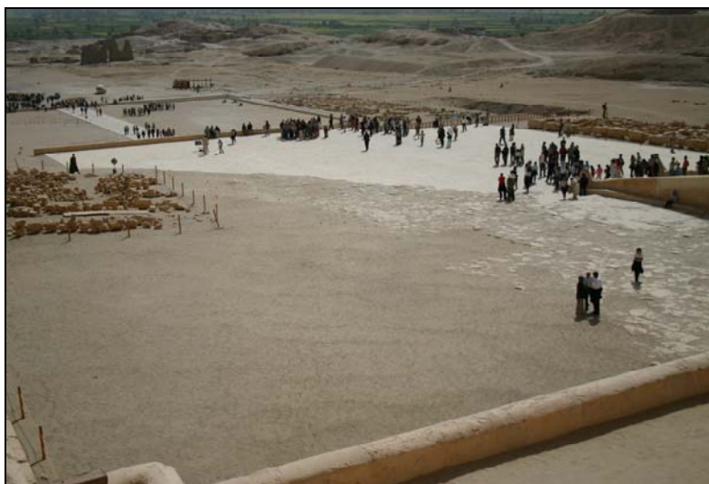
Fig. 4. Medium terrace of temple. One can see gray area of Esna shale removed during preparation for construction of temple. Artificially constructed part of terrace composed of block removed from upper terrace and covered with limestone plates seen deeper on photo
