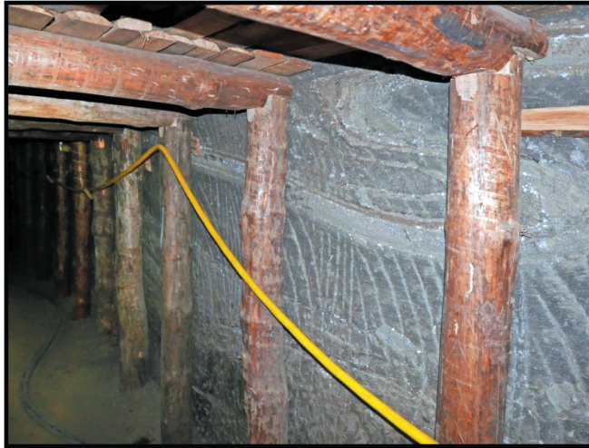
Fig. 2. Baum longitudinal. The area of the planned shaft. Exposure of bronze salts with intergrowths of anhydrite claystones. As of July 2017 [4]
