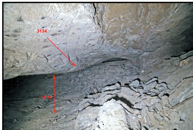
Fig. 4. Baum Chamber. State as of November 2018 [4]
