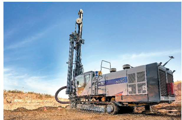
Fig. 6. Furukawa rig in the process of drilling
