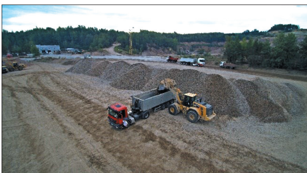
Fig. 16. Loading on a yard with a CAT 972M loader
