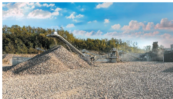
Fig. 14. Mineral aggregates production plant
