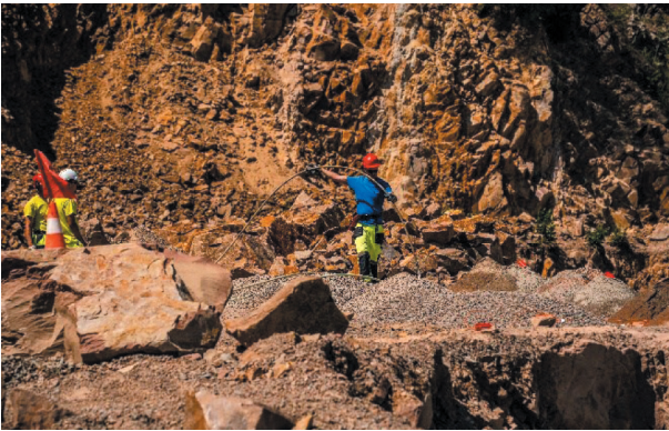
Fig. 8. Blasting works performed by SSE
