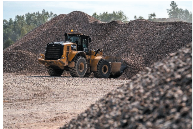
Fig. 17. Loaders during cleaning works
