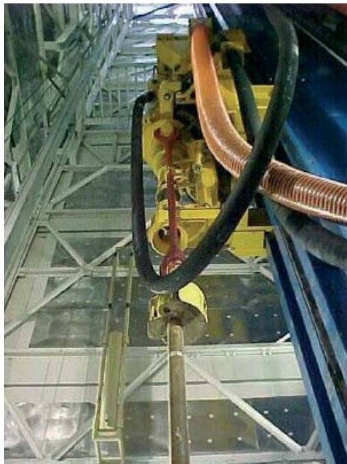
Fig. 2. The pipe handling machine
